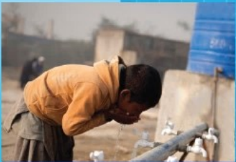
Rural Area Piping
