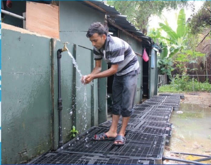
Potable Water Supply Pipeline
